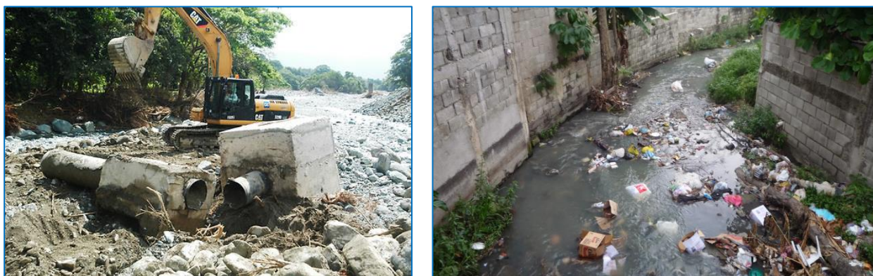
Figure 3: Water Sources Contamination in San Cristobal
