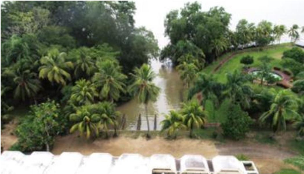
Figure 37: Existing Condition of Outflow Area
