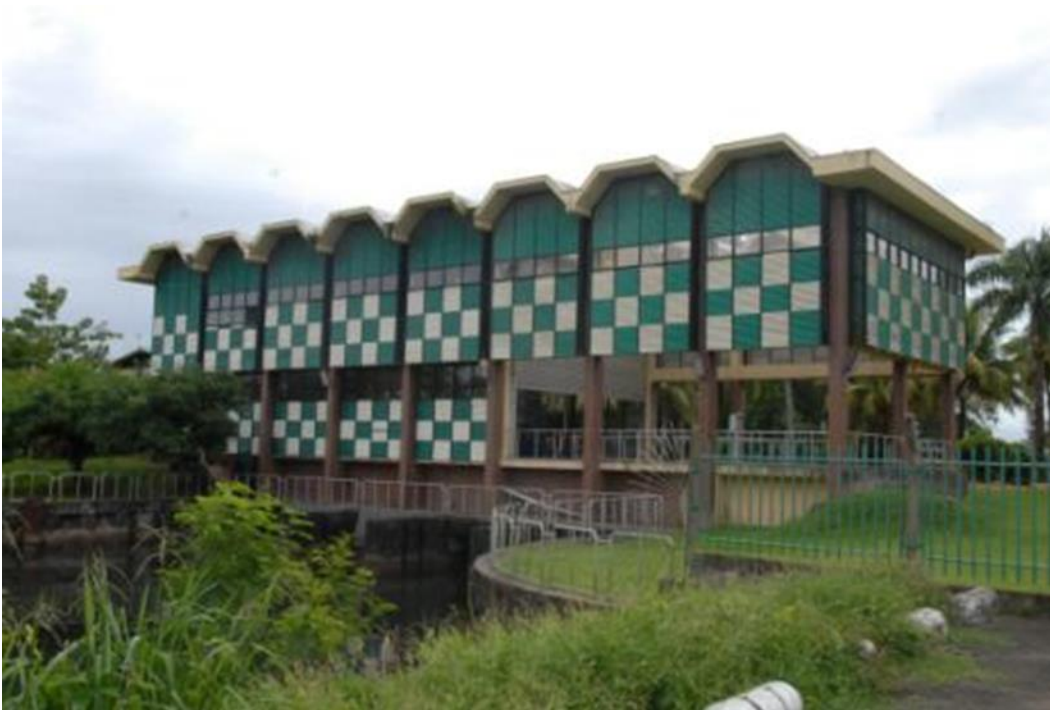
Figure 36: Existing Pump House
