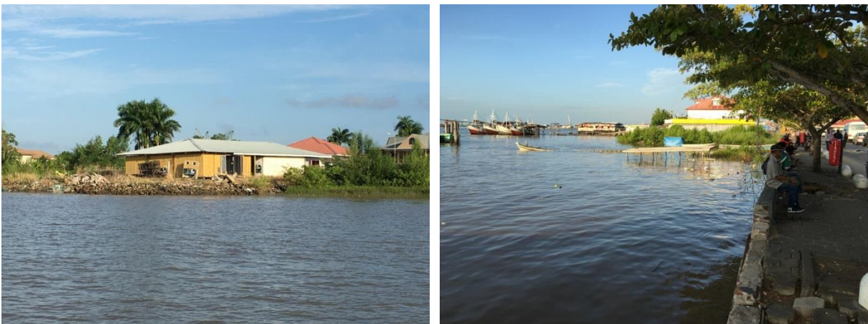
Figure 4: Examples of existing Flood Defences along the left bank of the Suriname River (Source: IDB, 2016).
