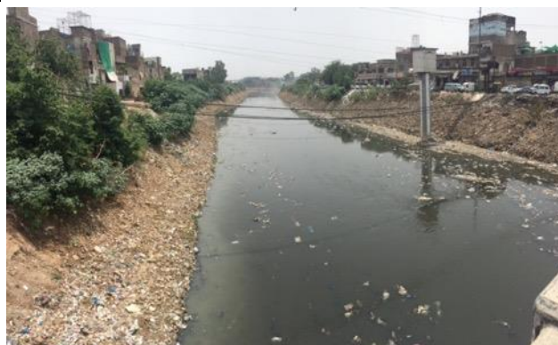
Figure 9: Lai Nallah in Rawalpindi
