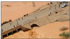
Plate 1. Air plane view showing flash flood damage of Sharg Alneel area, Khartoum City. Sudan (August 2013)
