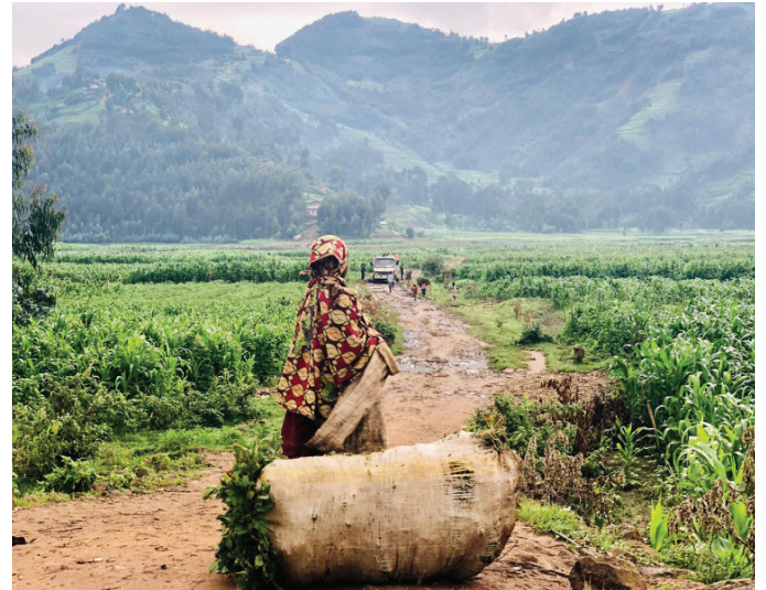
Cleaning drainage channels to reduce sediment in water flow and restore lowland farmland of Mugogo, Rwanda. Project implemented by the Rwanda Ministry of Environment. (Photo by Adaptation Fund)
