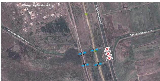
Figure 20: Detail of crossing "2" where the pipes under the irrigation channel are collapsed
