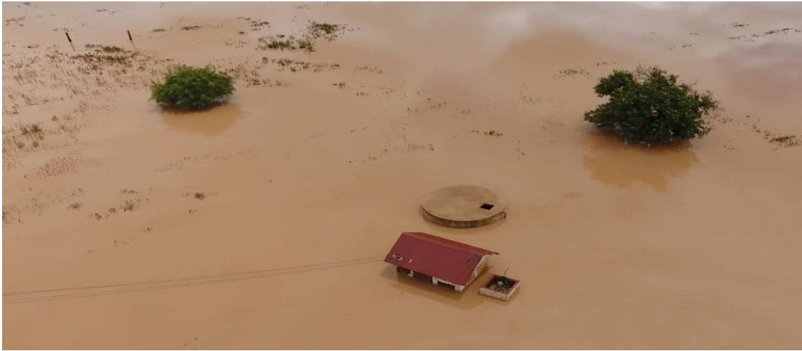
Figure 3: Flooded pump house in the Mbuga area at Mtanana village
