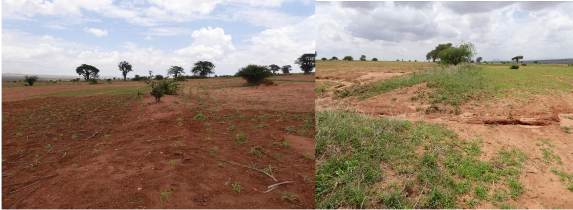
Figure7: A bund being farmed (left side) and Spot failure along a bund Right side) (Source: Field survey during the preliminary project design)
