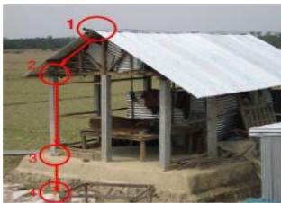
Figure 3-1: Strengthening of rural houses using ties (Source: IFRC BD Shelter Volunteer Training after cyclone Sidr)
