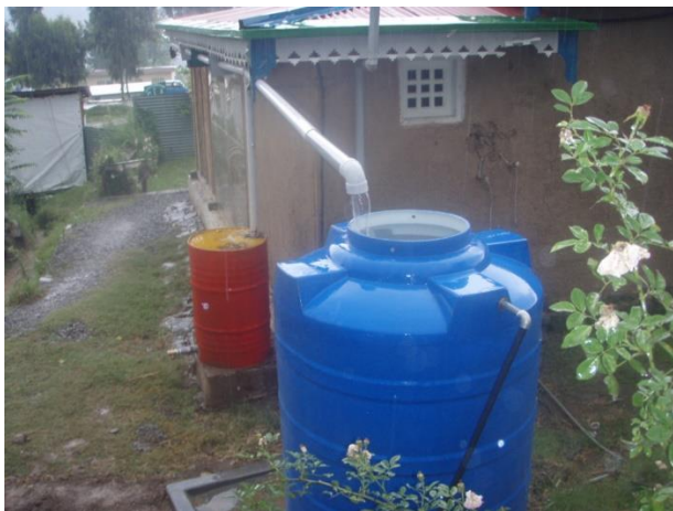
Figure 1: A household level rainwater harvesting setup installed by UNHABITAT in the earthquake affected areas of Pakistan
