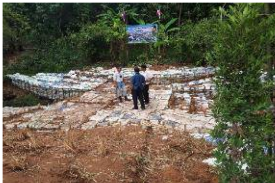
Living Check Dam construction
