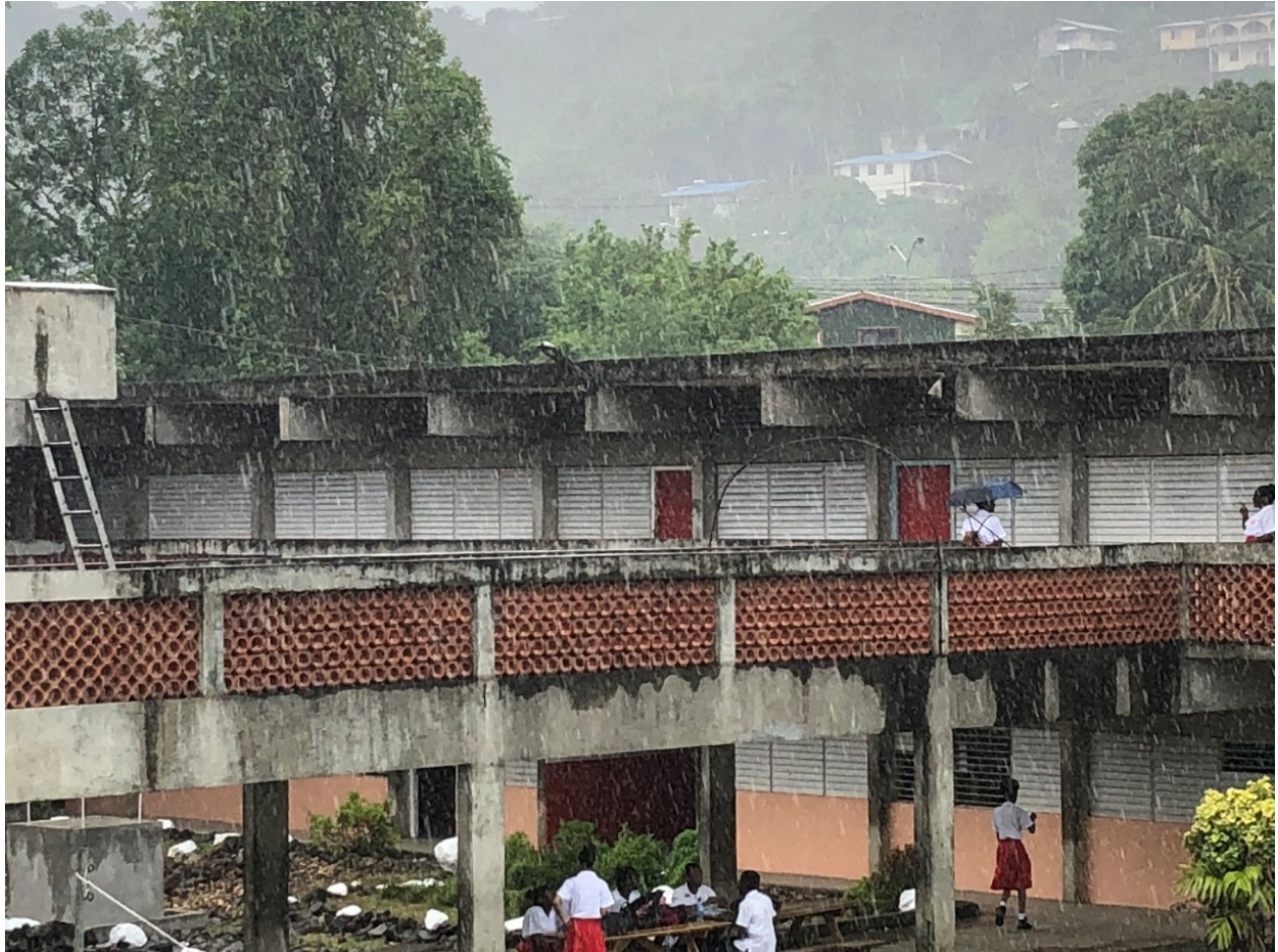
Photo of a public school in Saint Lucia
