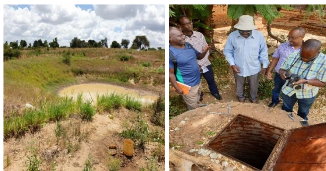
Figure 12: Shallow water basin and deep ground water tank in Kitui site in Kenya.
