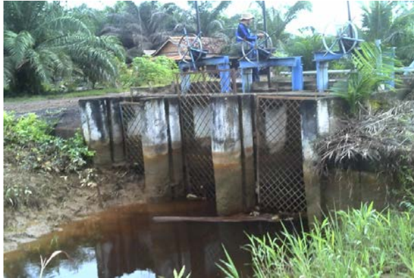
Figure A17: Non-functioning irrigation gate in Rejosari Village, Muara Sugihan Sub-district
