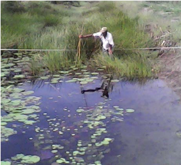
Figure A19: Non-maintained irrigation channels in Daya Murni Village, Muara Sugihan Sub-district
