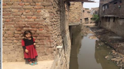
Figure 11: Drainage channels closed-in by houses and filled with waste in target communities in Rawalpindi – flood levels reach four meters above the channel banks, which is the 2 nd floor of houses.
