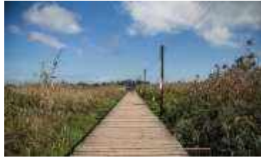
Image I.2-4: Wooden Bridge in Bandar-e-Kishahr
