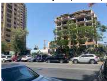
Image A.1-1: Housing under construction in Baku city center
