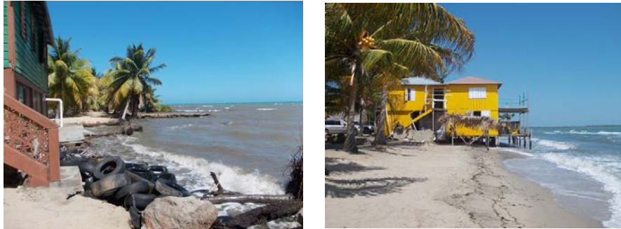
Figure 3. Images depicting erosion in Dangriga and Hopkins, respectively (NCCO)
