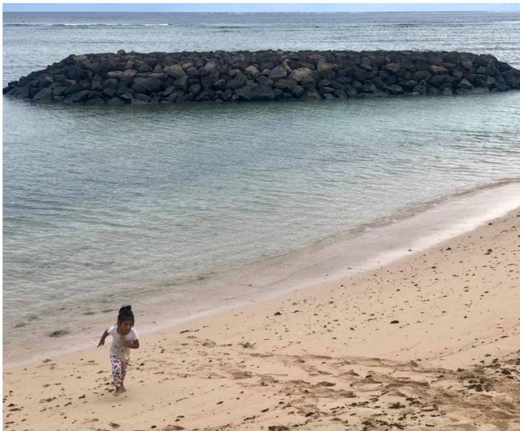
Picture 2: Wave breaker to avoid coastal erosion in Savai'i
