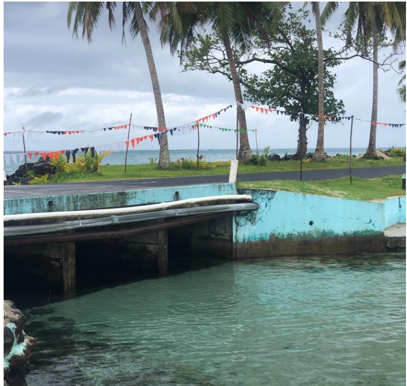
Picture 1: Asaga project revetment wall close to mangrove habitat
