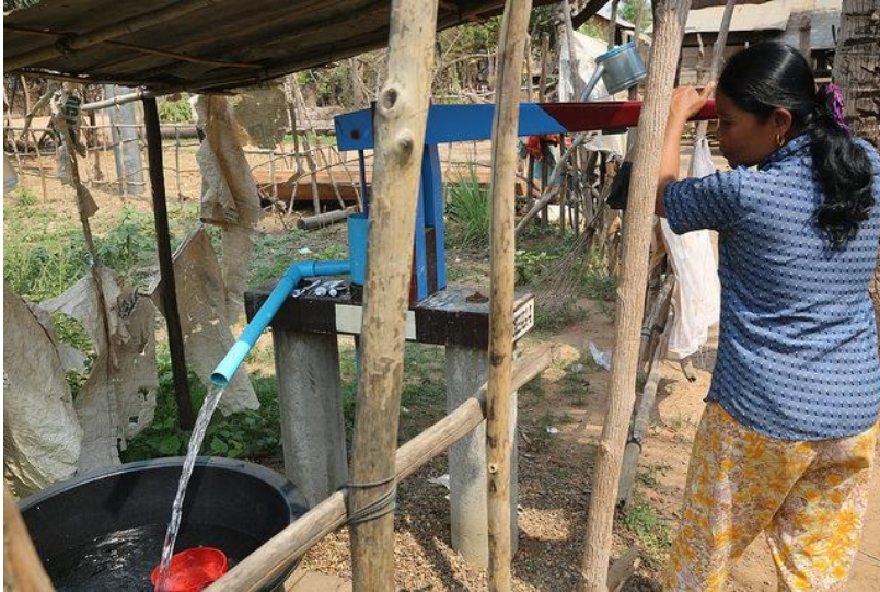
Figure 4: Water pump constructed in Skor Krouch CPA
