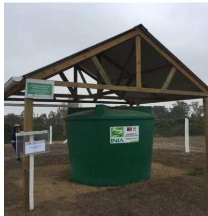
Picture 4: Rainwater collection tank with a capacity of 5,400 liters is also provided by the project to beneficiaries.
