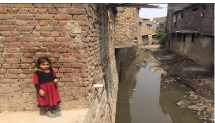
Figure 11: Drainage channels closed-in by houses and filled with waste in target communities in Rawalpindi – flood levels reach four meters above the channel banks, which is the 2 nd floor of houses.
