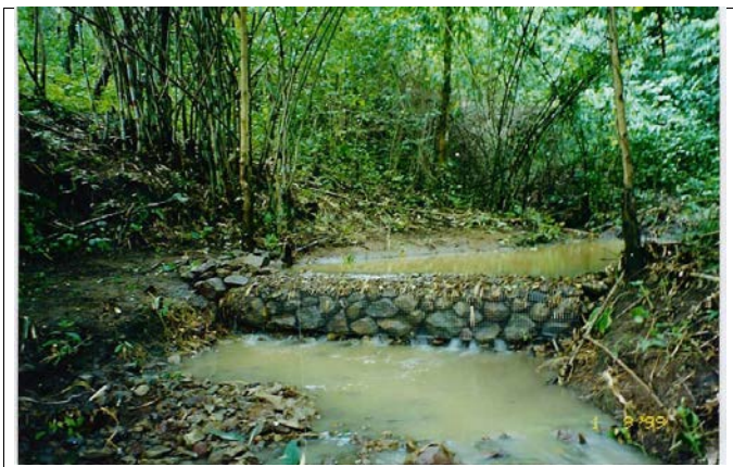
Figure 19: Example of a rehabilitated weir.
