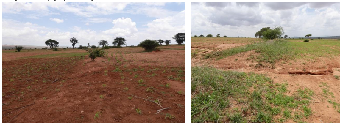
Figure 6: A bund being farmed (left side) and Spot failure along a bund Right side) (Source: Field survey during the preliminary project design)
