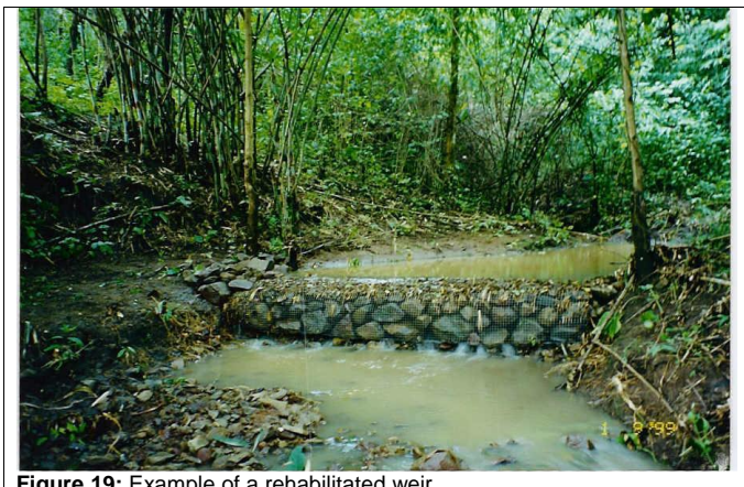
Figure 19: Example of a rehabilitated weir.
