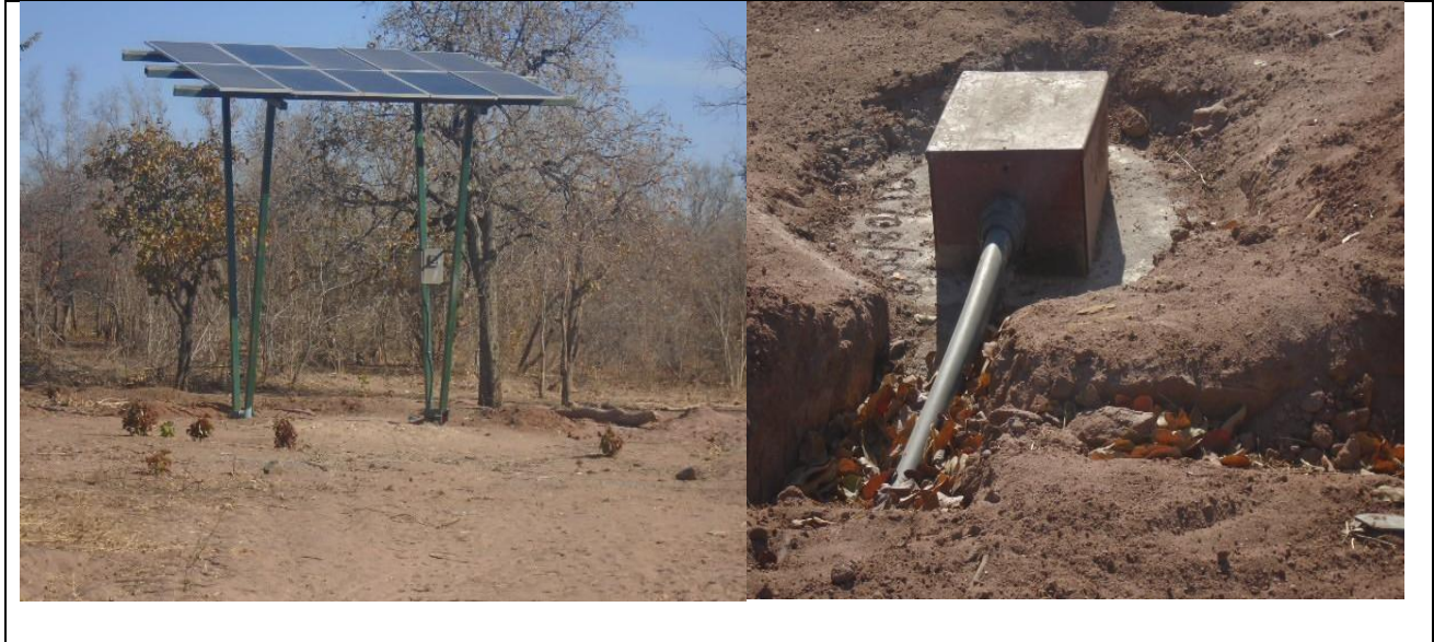
Figure 40: Pictures of solar powered borehole drilled by ZRBF in Binga Ward 25
