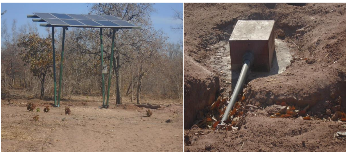
Figure 54 Pictures of solar powered borehole drilled by ZRBF in Binga Ward 25
