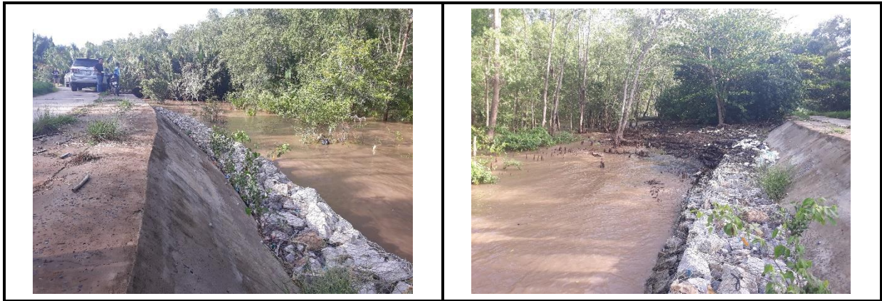
Figure 5.1 Installed concrete dike in Long Hoa commune
