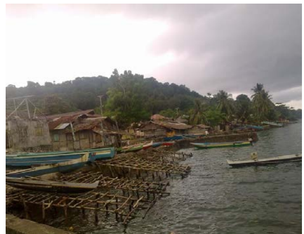
Figure 6. Fishermen built stilt structure for docking their boats due to the increase of sea water level
