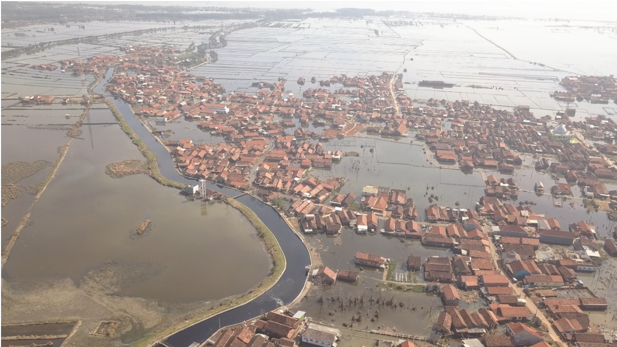
Figure 4. Severe Flooding in Pekalongan City
