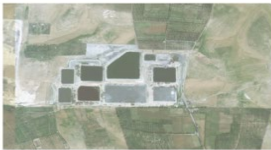
Waste water treatment plant Akaidr
