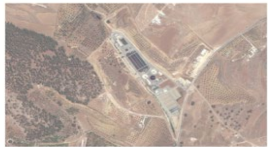
Waste water treatment plant Maered
