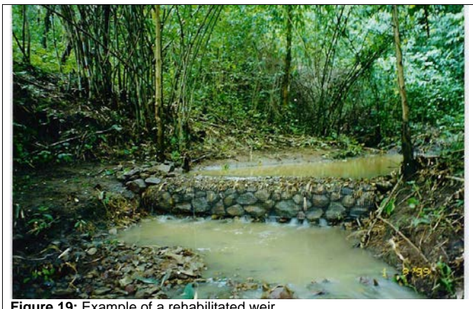
Figure 19: Example of a rehabilitated weir.
