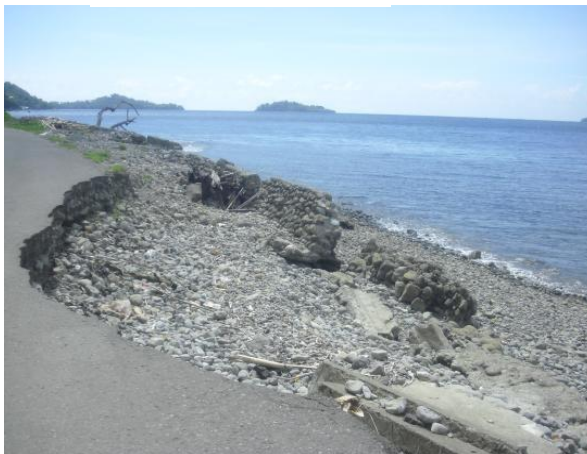
Figure 5. The impact of tidal waves and abrasion in the form of damage to road infrastructure and breakwater walls due to tidal waves
