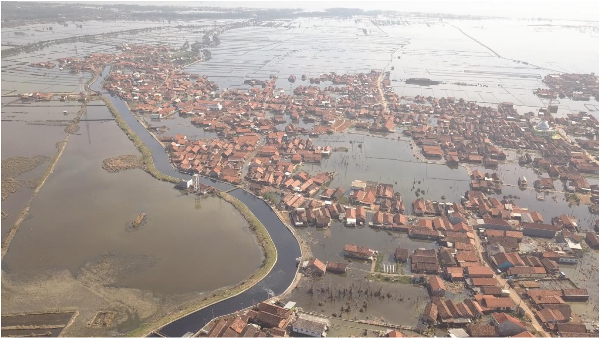
Figure 4. Severe Flooding in Pekalongan City
