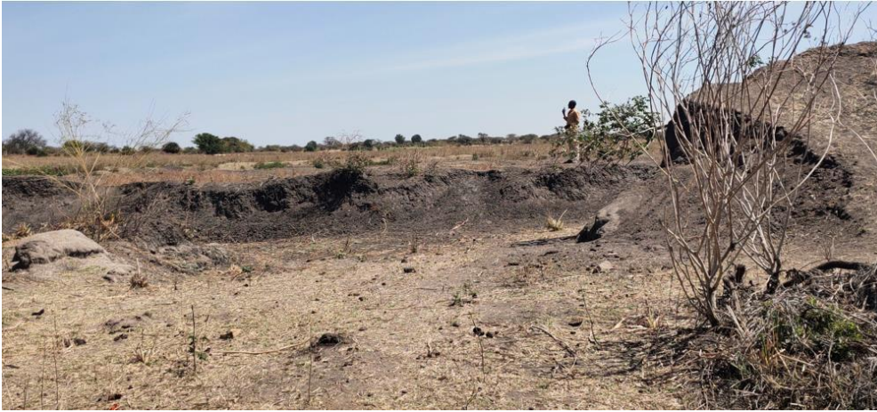
Annex Figure 2: Broken dyke and spillway of the dam at Nguriti, hence low water storage capacity of the dam. Siltation has also filled the dam leading into low water storage capacity.
