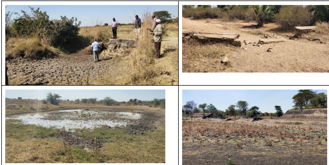
Figure 10: Broken embankment and spillway of dams as observed during field survey and stakeholders’ consultation exercise in June 2019 by project team. These water-harvesting dams have become shallow due to high siltation and can barely store rainwater during dry season for 2 months only.
