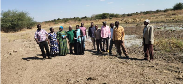
Annex Figure 11. Kabudyo dam in Ntoba village had broken embankment with extreme siltation such that has lost water holding capacity.
