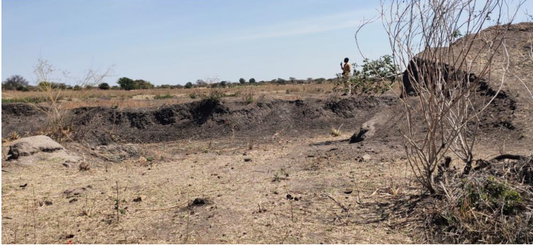
Annex Figure 2: Broken dyke and spillway of the dam at Nguriti, hence low water storage capacity of the dam. Siltation has also filled the dam leading into low water storage capacity.
