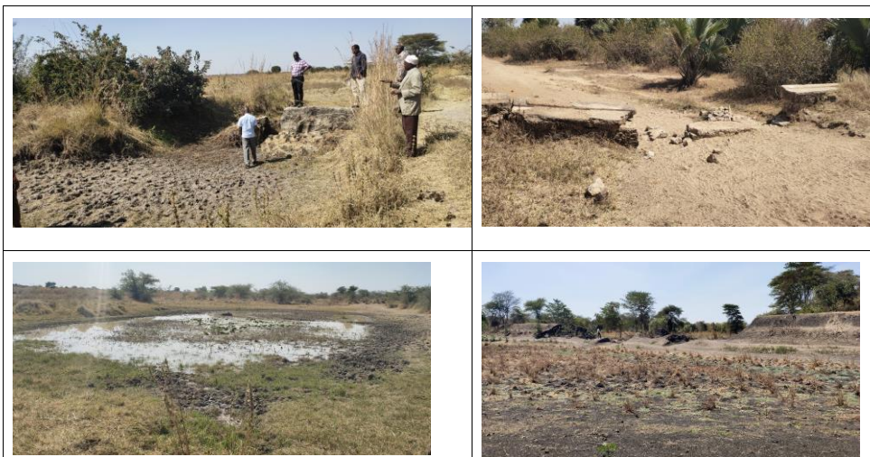
Figure 10: Broken embankment and spillway of dams as observed during field survey and stakeholders’ consultation exercise in June 2019 by project team. These water-harvesting dams have become shallow due to high siltation and can barely store rainwater during dry season for 2 months only.
