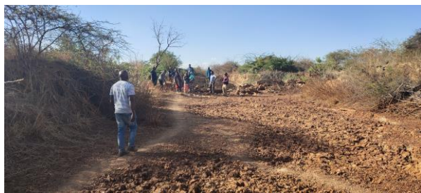
Annex Figure 7 Broken embankment and spillway of the dam at Mtitaa causing low water storage capacity of the dam.
