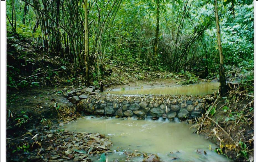
Figure 19: Example of a rehabilitated weir.
