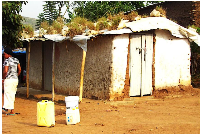
Figure 3. 'Roof Top Gardens', a '3 in 1 climate change adaptation measure' to hold roofs against strong winds, moderate high day-time temperatures, and grow vegetables as food security
