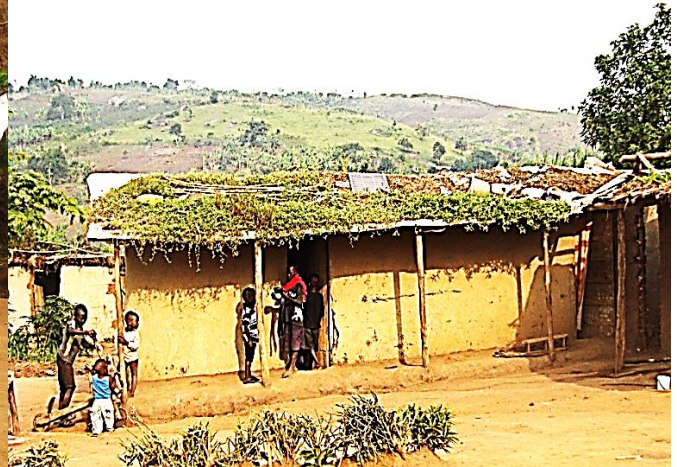
Figure 13: Solar Panel as an alternative energy source
