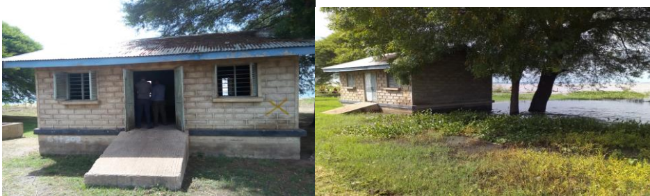
Figure 7: The observed effect the recent rise in Lake Victoria water levels to the pump houses at Kasahunga, water sources. The sources was designed in 1970s without integration of climate change issues in during the design. The proposed intervention under output 1.1 avoids such mistake, and considers projected /future climate events under various scenarios including optimistic ones. The photo on the left hand side was taken in July 2019 before the rise of lake water levels while the photo on the right hand was taken in February 2020 after the rise of Lake water levels due to floods and extreme precipitation events.
