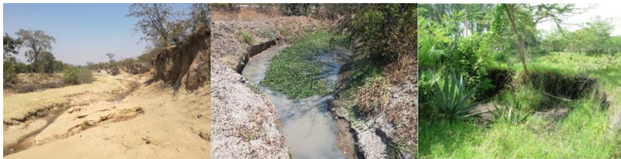
Figure 16 Gullies in Binga and Buhera and some gully protection measures in use in Zimbabwe using sissal
