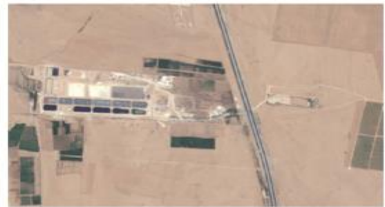
Waste water treatment plant Mafraq
