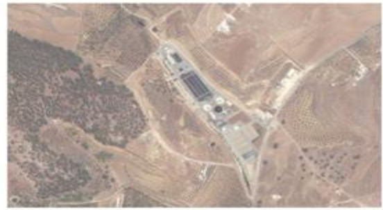
Waste water treatment plant Maered
