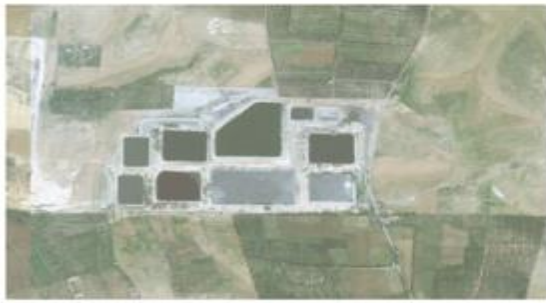
Waste water treatment plant Akaidr
