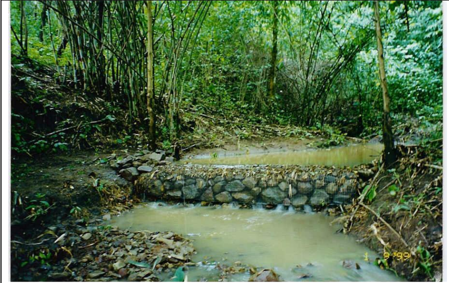
Figure 19: Example of a rehabilitated weir.
