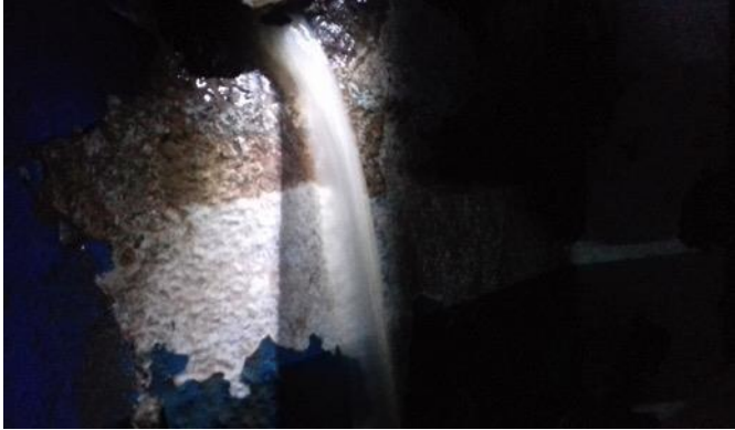
Basement of the 12 th apartment of Khilchin hothon – flood water and ground-water penetrating from the walls and floors leading to power cut restriction of 670 households Photo (UN-Habitat June 2017)
