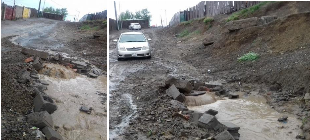
Flooding of main road sinkhole constructed by the Geodetic Water Facility Office of the Housing Authority (UN-Habitat June 2017)
