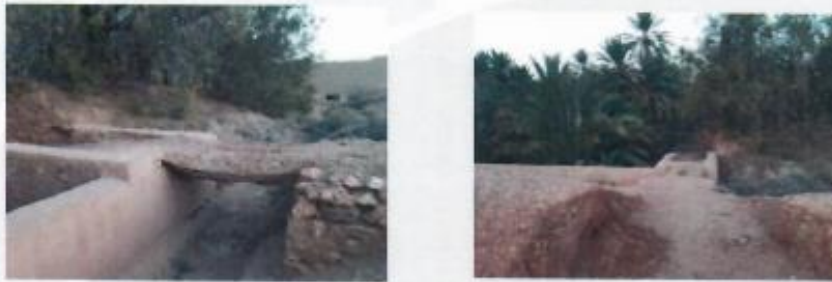
State of the walkways accessing the palm grove ravaged by fire.
