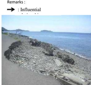
**Figure 5.** The impact of tidal waves and abrasion in the form of damage to road infrastructure and Embankment walls due to tidal waves
