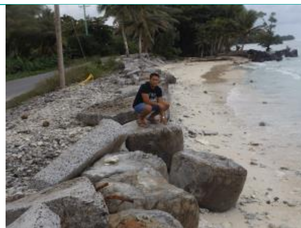
Mosral section of Malem road. mass concrete bags, loose boulders, and broken concrete, placed randomly to reduce surge impact and prevent wave overtopping and erosion of road (photo credit: Simpson Abraham, 2015)
