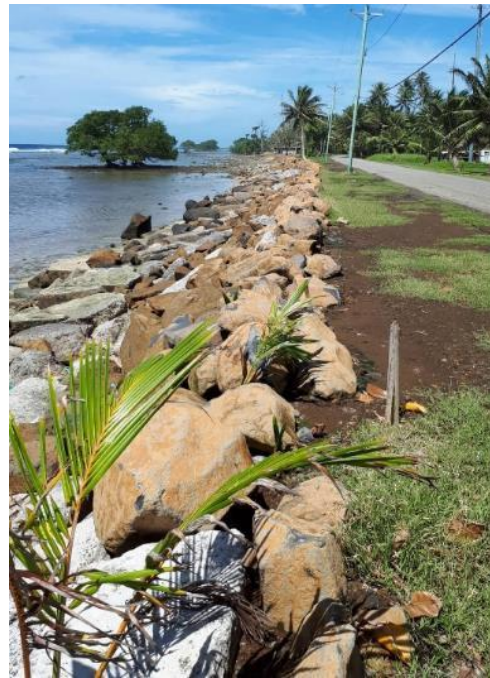
Figure 11: Existing emergency coastal defence works at Mosral (left) and Paal (right)
