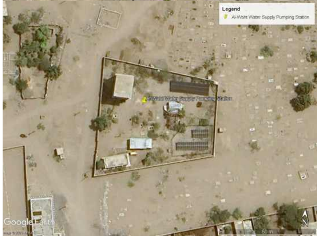
Figure 61 Al-Hawtah city and water supply pumping station
