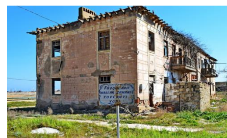
Image A.2-1: Housing situation on Pirallahi Island 19
