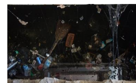
Image A.2-4: Basements of some residential buildings in Pirallahi district are flooded 22
