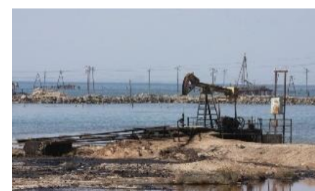
Image A.2-3: The site has been area of extensive oil exploitation and left with many dilapidated equipment 21
