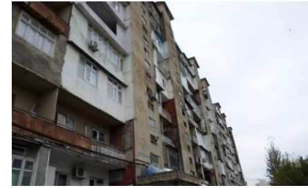
Image A.3-1: Typical multi-story building in Neftchala without access to water during drought (source: Anar Valiyev)
