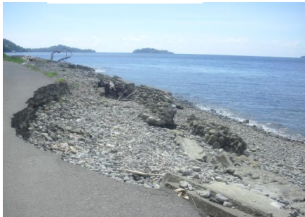
Figure 5. The impact of tidal waves and abrasion in the form of damage to road infrastructure and Embankment walls due to tidal waves
