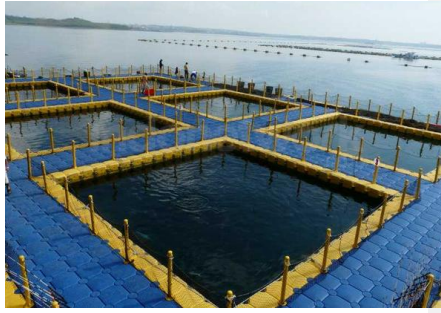
Picture Source : coolboxindonesia.com Example of modern floating cube cage "interlocking system" made of HDPE materials
