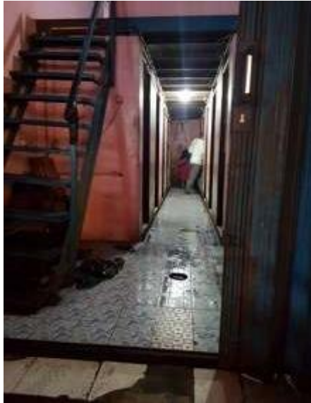
Figure 2. Sanitation facilities at Pasar Segiri with toilets with limited space for women with children.
