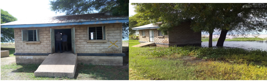
Figure 9: The observed effect the recent rise in Lake Victoria water levels to the pump houses at Kasahunga, water sources. The sources were designed in 1970s without integration of climate change issues in during the design. The proposed intervention under output 1.1 avoids such mistake, and considers projected /future climate events under various scenarios including optimistic ones. The photo on the left-hand side was taken in July 2019 before the rise of lake water levels while the photo on the right hand was taken in February 2020 after the rise of Lake water levels due to floods and extreme precipitation events.
