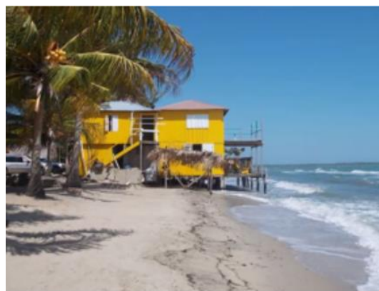
House being consumed by the approaching sea due to erosion in Belize.
