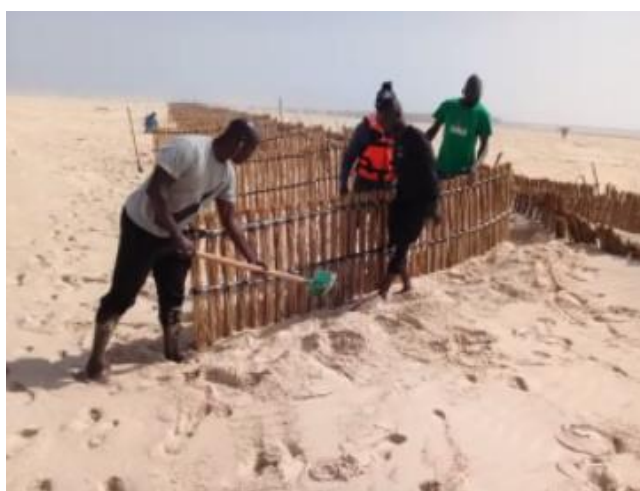
Local community workers install sand retention barrier near Saly.
