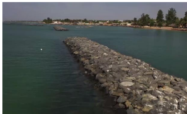
Dike constructed near Joal.
