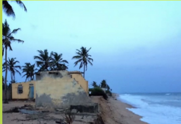
House impacted by beach erosion. photo CSE
