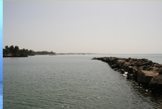
Barriers such as these help prevent extreme erosion. photo CSE
